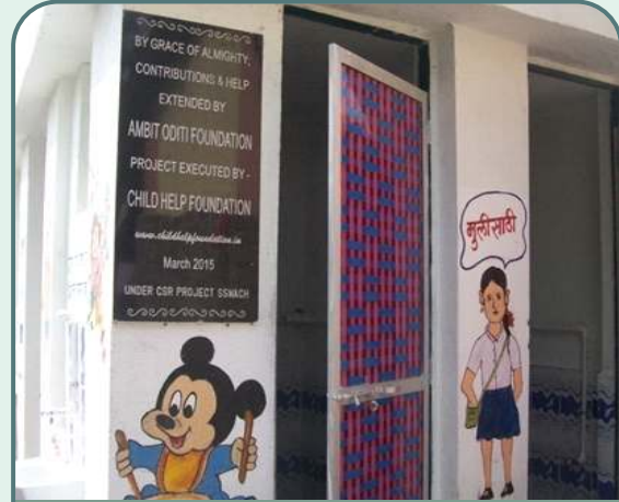
Front Side of the School Toilet
